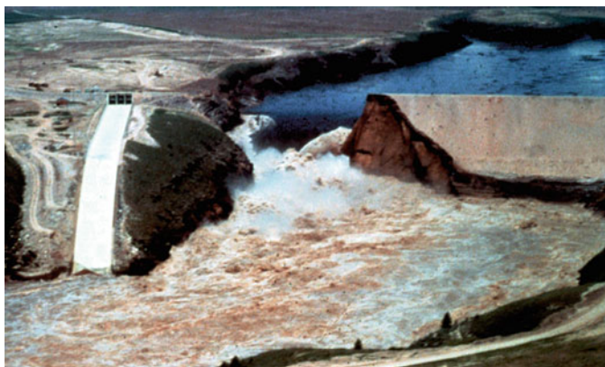
Fig. 2.9 Degradation of dam (due to pressure of water) and eventual failure
